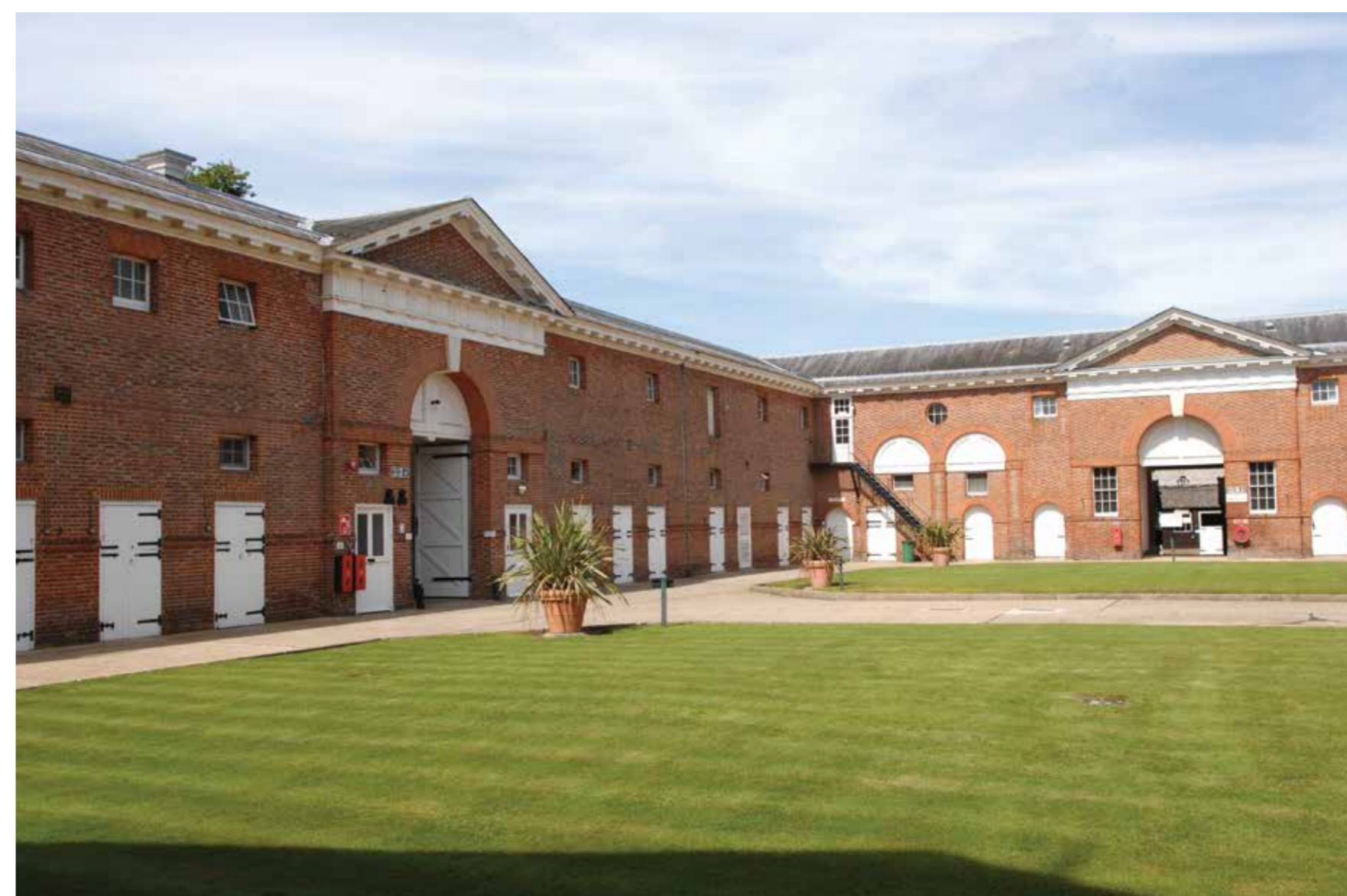
The brick courtyard of the Stables
